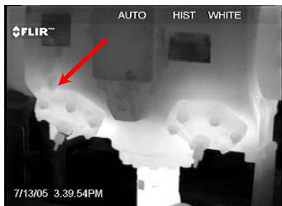
Figure 5a. Leak from LPG compressor left flange.
