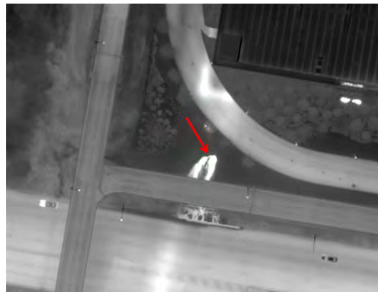
Figure 4b. Infrared image of a steam distribution line leaking liquid up, onto the ground surface.
