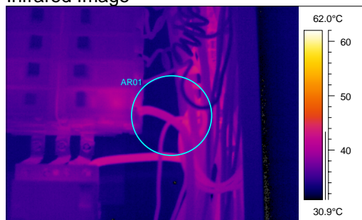
Figure 3: Post-repairs: The thermal pattern is uniform
