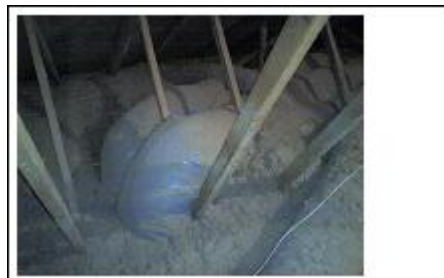
Figure 14b. Visual image of duct
